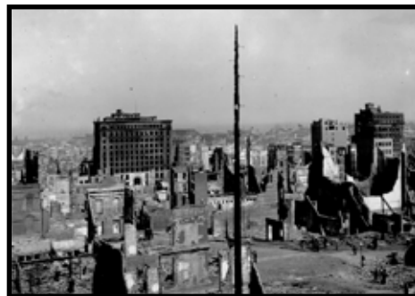
San Francisco earthquake, 1906
