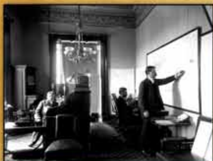
White House Communications Room, 1898
