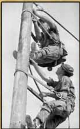
Cable repair, Vietnam
