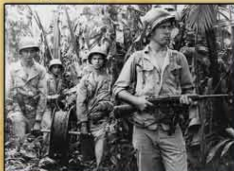
Laying wire at Bougainville Island in the South Pacific, 1943
