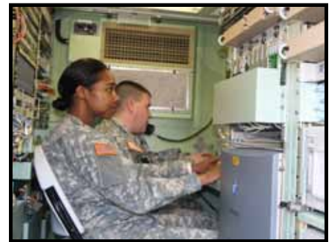
Joint Network Node shelter
