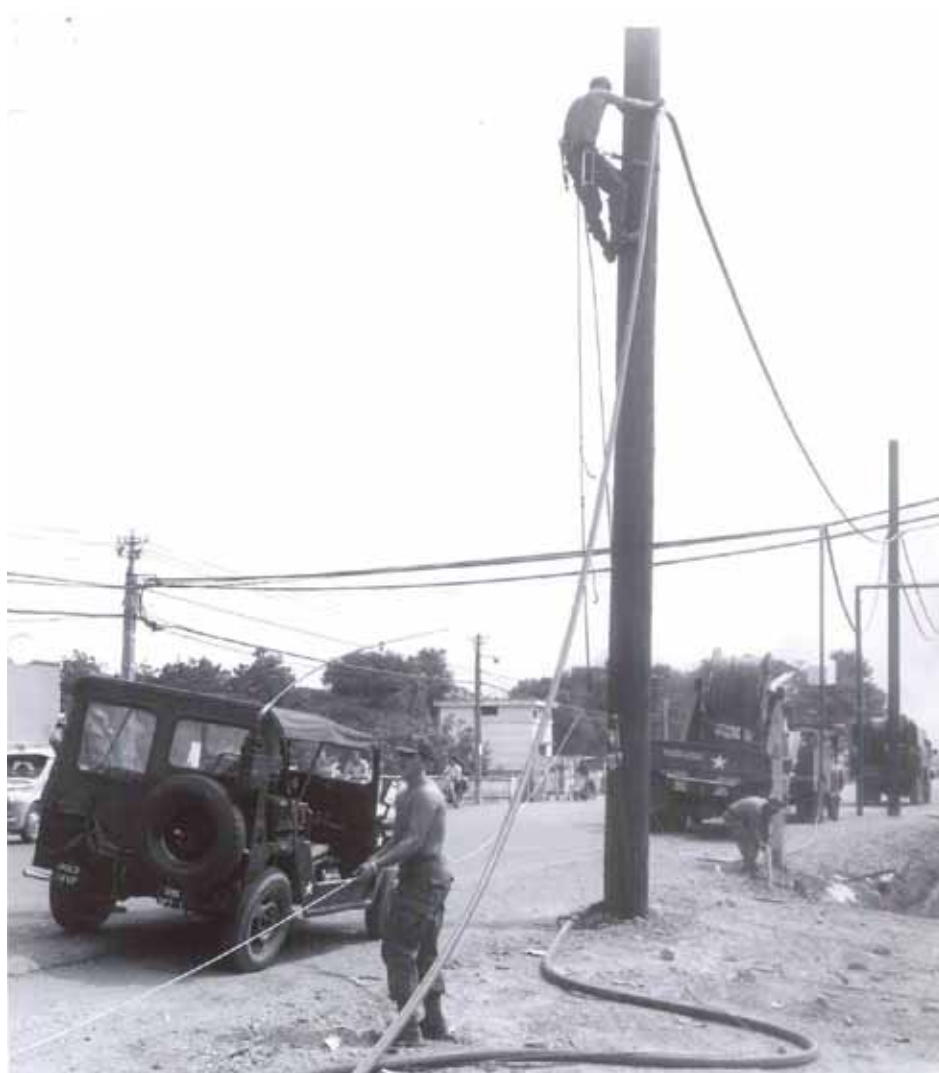
Cable dawgs of U.S. Army STRATCOM's 69th Signal Battalion effect communications cable repairs following a fire fight on Plantation Road in Saigon, South Vietnam in April 1969
