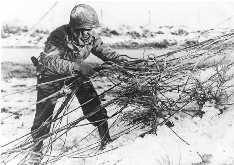
A Signal lineman working in the European theater in 1945
